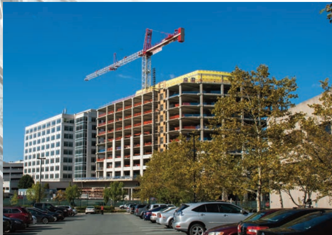
Choice International Hotels' new headquarters under construction.
